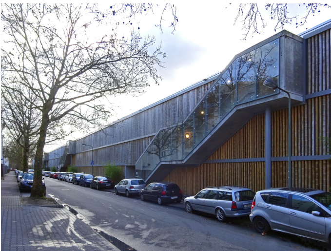
Quartiersgarage in Praunheim
